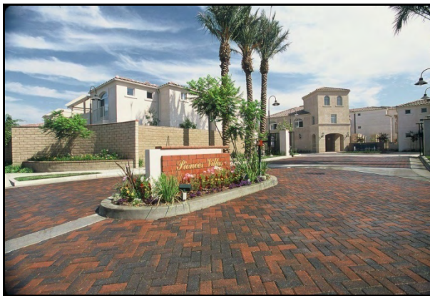
Main entrance with lush landscaping
